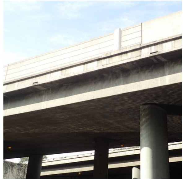
Figure 2-5. Storm Drain Outfalls from I-5 Freeway Hollenbeck Park Lake Rehabilitation and Stormwater Management
