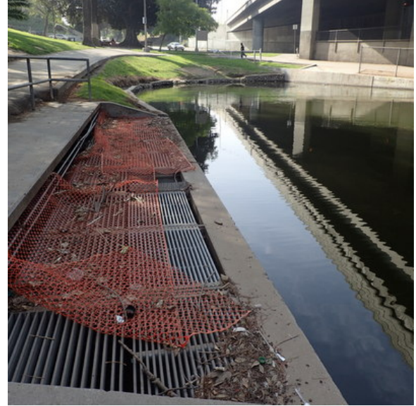
Figure 2-3. Southern Outlet Structure Hollenbeck Park Lake Rehabilitation and Stormwater Management
