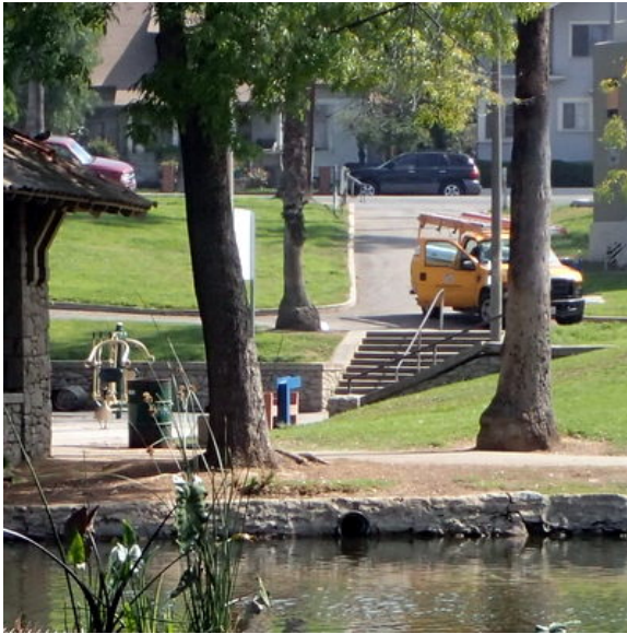
Figure 2-4. Storm Drain Outfall to Lake Hollenbeck Park Lake Rehabilitation and Stormwater Management
