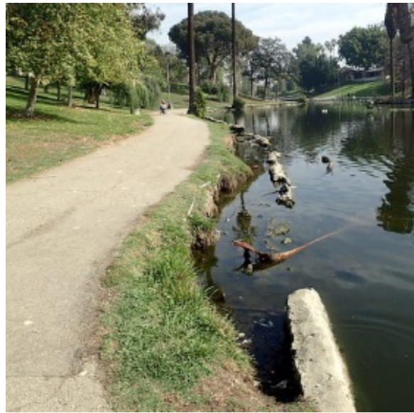
Figure 2-7-D. Lakeside Erosion Hollenbeck Park Lake Rehabilitation and Stormwater Management
