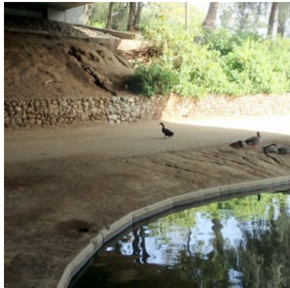
Figure 2-7-B. Erosion Rills on Abutment and Lake Edge Hollenbeck Park Lake Rehabilitation and Stormwater Management
