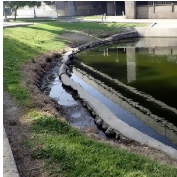
Figure 2-7-P. Lakeside Erosion Hollenbeck Park Lake Rehabilitation and Stormwater Management
